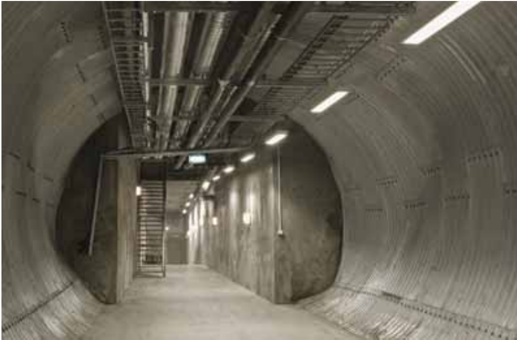
Overgang Svalbardrør/portal- bygg. Connection between “Svalbard tube” and portal building.
