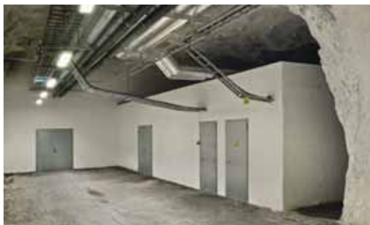
Servicebygget / The service building
